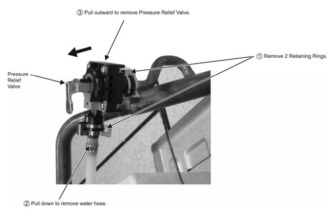
${\color{red} \underline{\Lambda}}$  When reinstall the water pipe, use grease or water at the joining.
