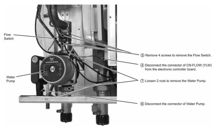
⚠ When reinstall the water pipe, use grease or water at the joining.
